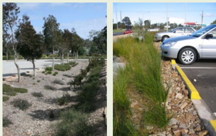
EXAMPLES OF DRAINAGE SWALE
