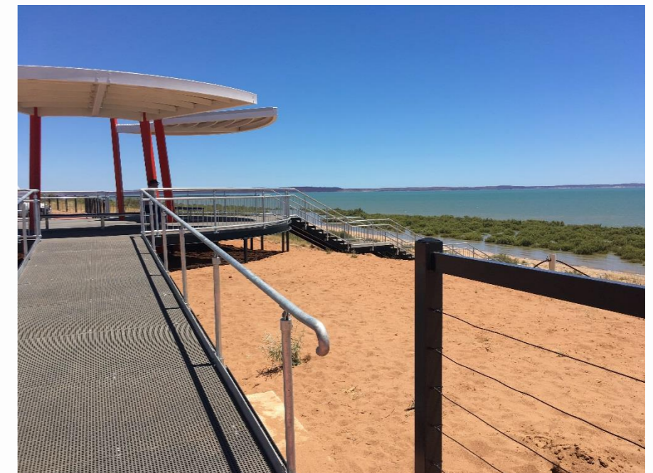
Figure 15 – Coastal Infrastructure at the Karratha Coastal Node.
