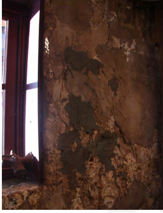
Cement patches to be removed. Source: TPG+PM 2017
