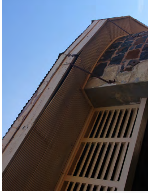
Damaged eaves and soffit. Source: TPG+PM 2017
