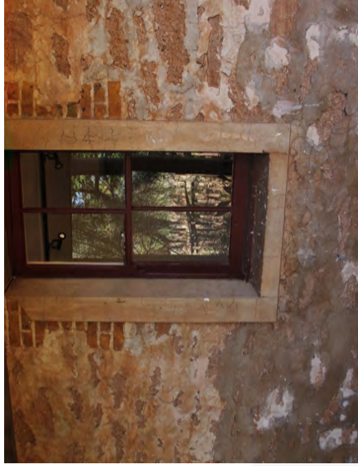
Efflorescence of salts due to cement render and rising damp. Source: TPG+PM 2017
