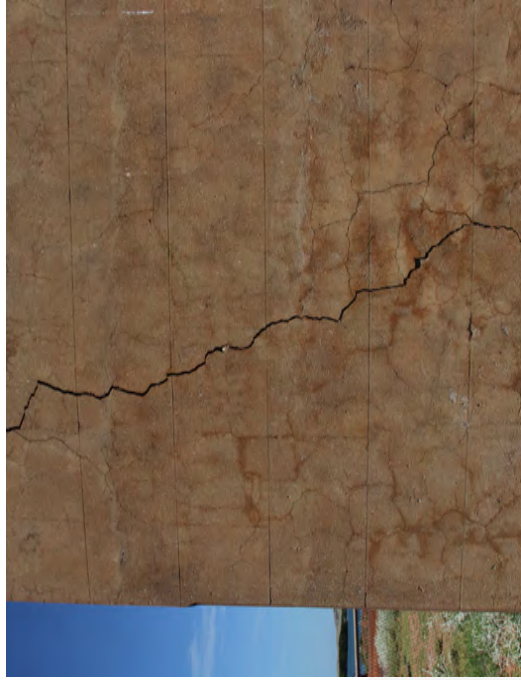
Major vertical crack. Source: TPG+PM 2017
