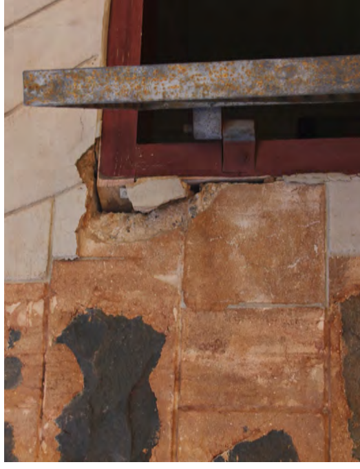
Repair to quoining. Source: TPG+PM 2017
