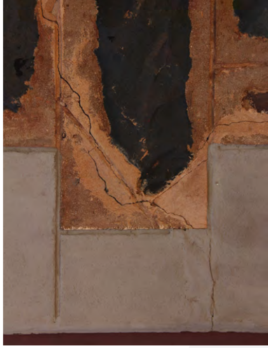
Hairline cracks throughout. Source: TPG+PM 2017
