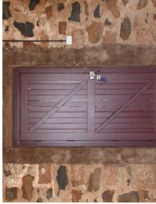
Efflorescence of salts due to cement mortar and the use of concrete to tie beams. Source: TPG+PM 2017
