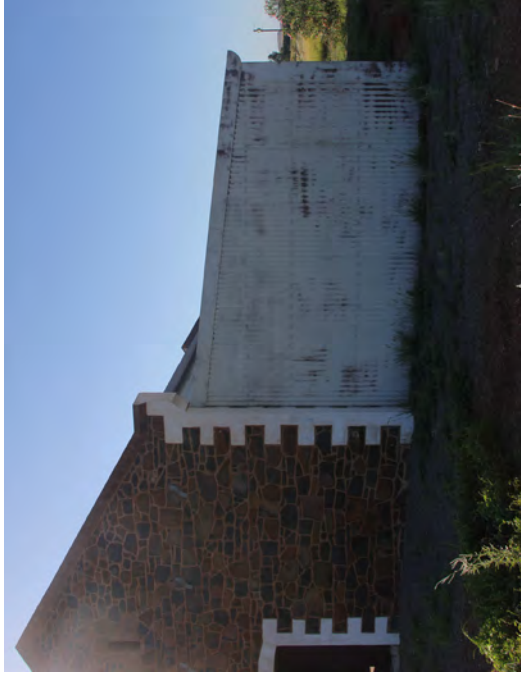
Galvanised iron lean-to annex. General rust and loose paint. Source: TPG+PM 2017
