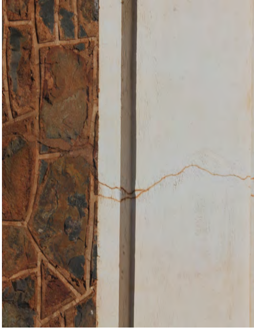
Hairline cracks throughout the walls. Source: TPG+PM 2017
