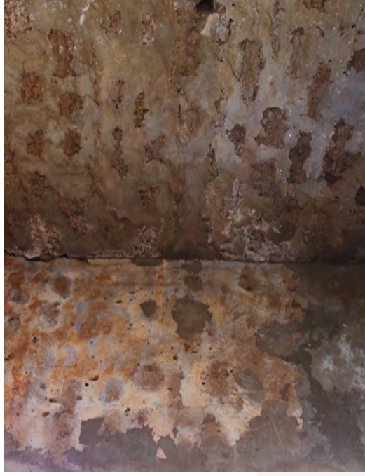
Efflorescence of salts due to cement mortar. Source: TPG+PM 2017
