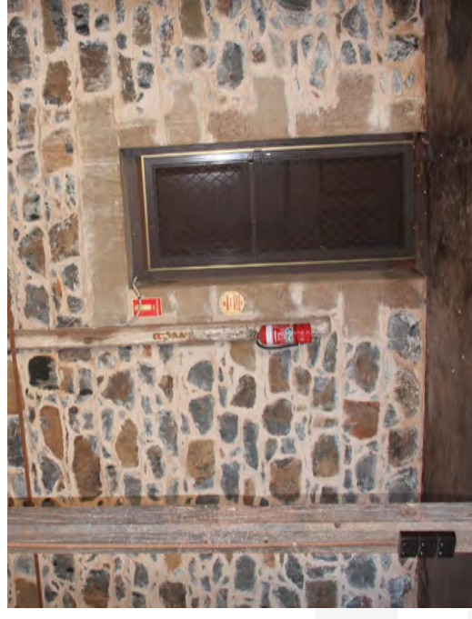
Cement pointing causing efflorescence of salts. Humidity patch over door. Source: TPG+PM 2017
