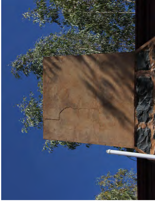
Major cracks to the chimney. Source: TPG+PM 2017
