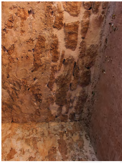
Friable original mortar on the wall base. Source: TPG+PM 2017
