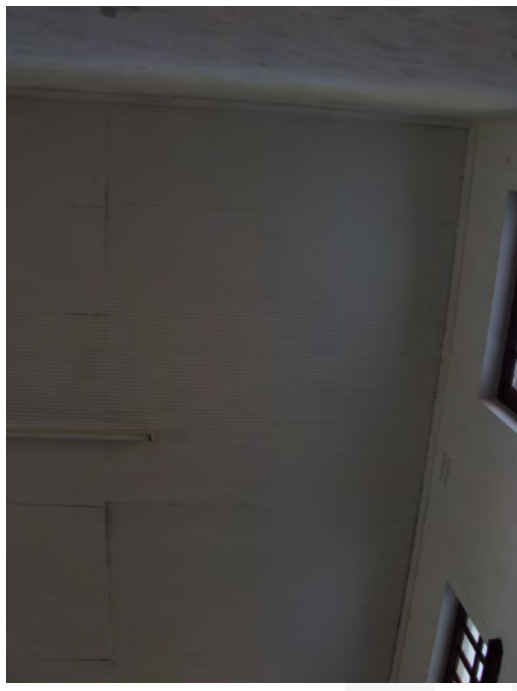
Pressed galvanised iron ceiling with loose sheets and signs of rust. Source: TPG+PM 2017
