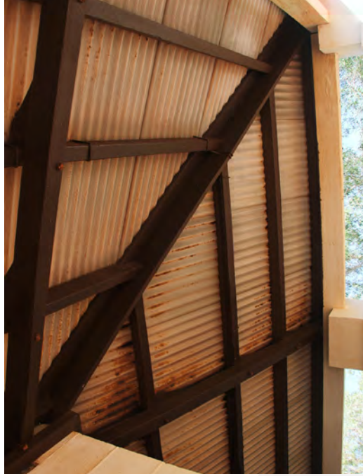
General rust on metal roof sheets. Source: TPG+PM 2017
