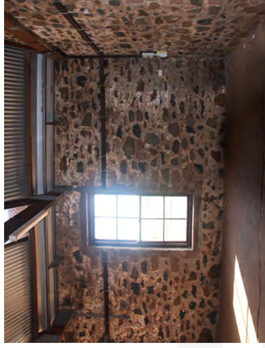
Store interiors with salts' efflorescence and cement mortar to bluestone walls. Source: TPG+PM 2017
