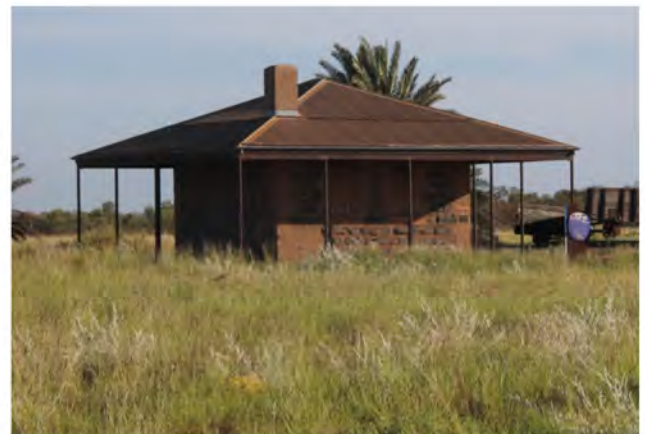
Figure 49. Cossack School in 2017 (Source: TPG).
