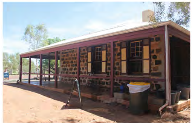
Figure 20. Police Quarters in 2017 (Source: TPG, 2017).
