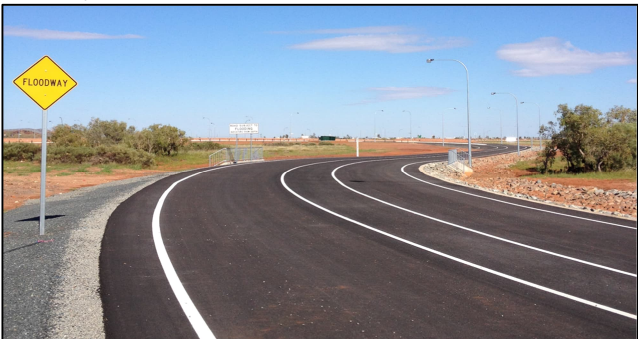
Figure 10 – Existing Prancing Avenue (Near Left-in off Madigan Road)
