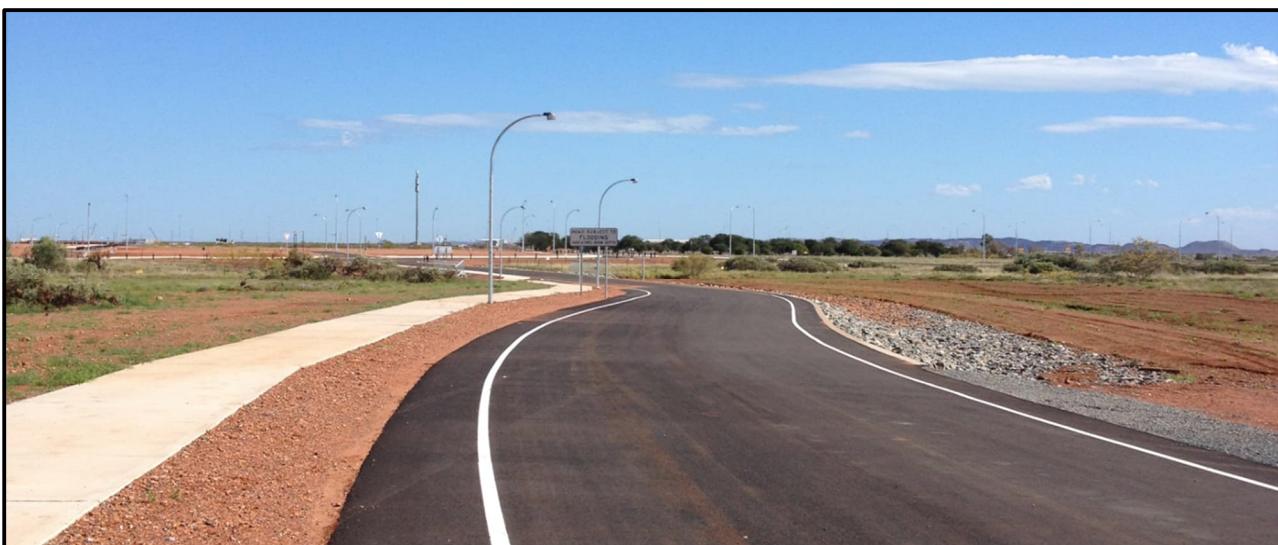
Figure 11 – Existing Gardugarli Drive (Full access weather crossing across Madigan Creek)
