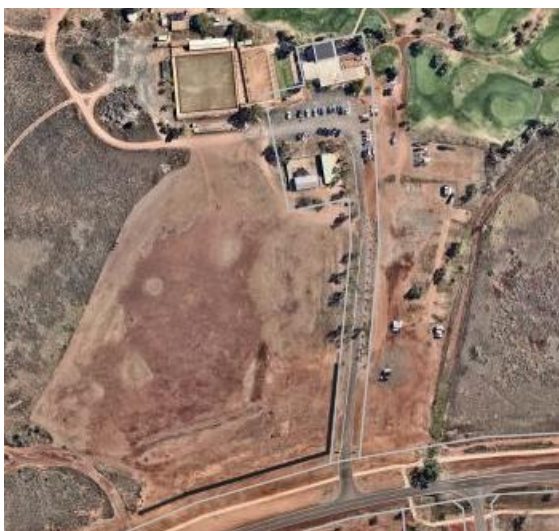
Figure 1 – Current Fencing Installation
