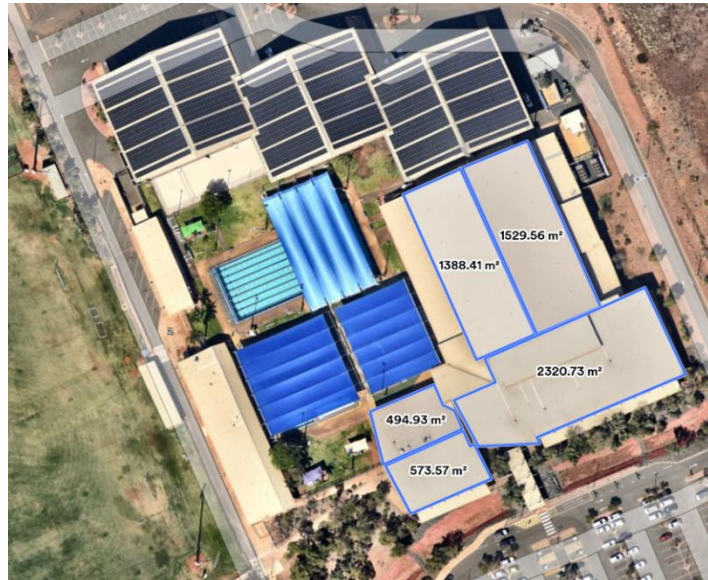
FIGURE 15: AERIAL VIEW AND AVAILABLE ROOFTOP AREA OF KARRATHA LEISUREPLEX
