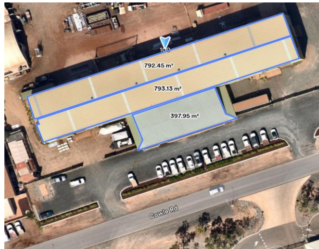
FIGURE 19: AERIAL VIEW AND AVAILABLE ROOFTOP AREA OF OPERATIONS CENTRE
