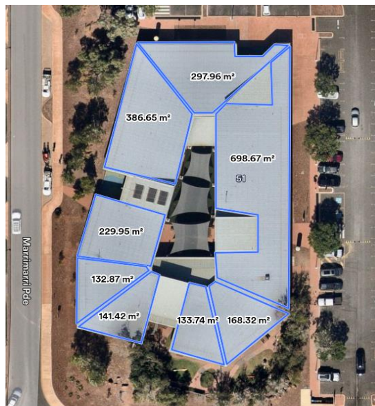
FIGURE 25: AERIAL VIEW AND AVAILABLE ROOFTOP AREA OF PAM BUCHANAN COMMUNITY CENTRE
