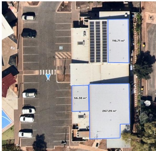
FIGURE 30: AERIAL VIEW AND AVAILABLE ROOFTOP AREA OF YOUTH SHED
