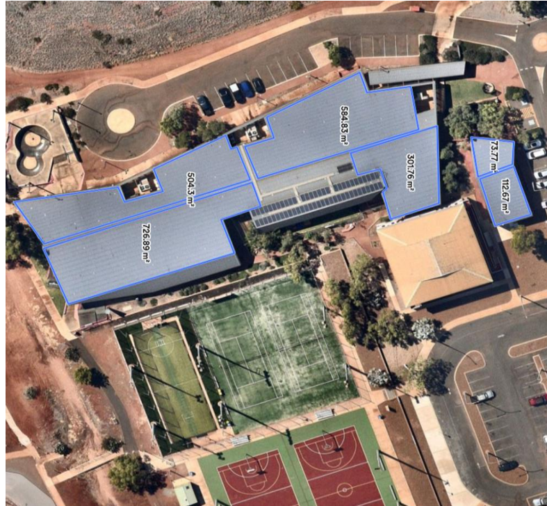
FIGURE 22: AERIAL VIEW AND AVAILABLE ROOFTOP AREA OF WICKHAM COMMUNITY CENTRE
